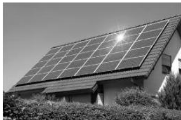
Figure 6. A solar photovoltaic cell array
